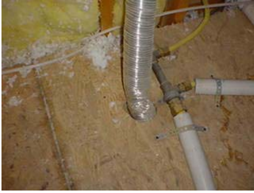
Flexible exhaust piping is damaged and should be repaired.
