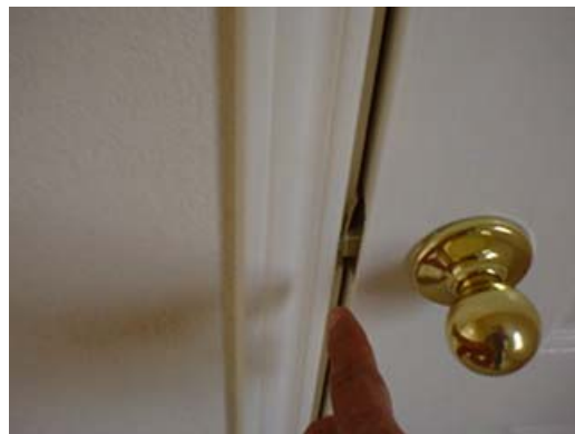
Door does not latch properly; minor adjustment to strike plate may be all that is needed.
