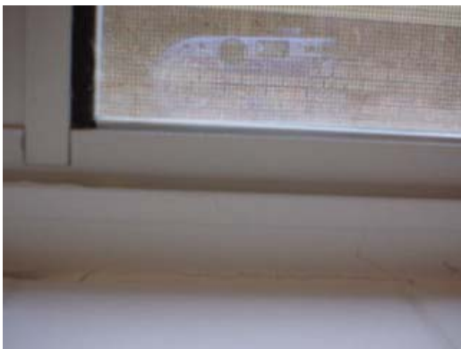
Window seal vulnerable to moisture intrusion monitor this area on a consistent basis and repair as needed.
