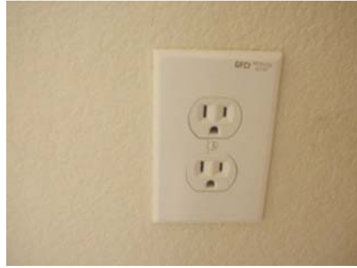
GFCI labeled receptacle in the garage did not respond favorable to the test and should be repaired.
