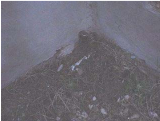
Erosion and exposed sprinkler system piping. Piping for sprinkler system should be at a minimum depth of 6".
