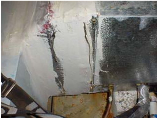
Seal cut here, should be repaired.
