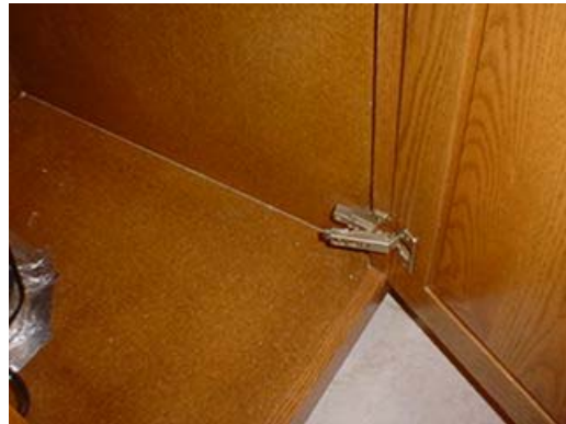
Cabinet door hinge needs repair
