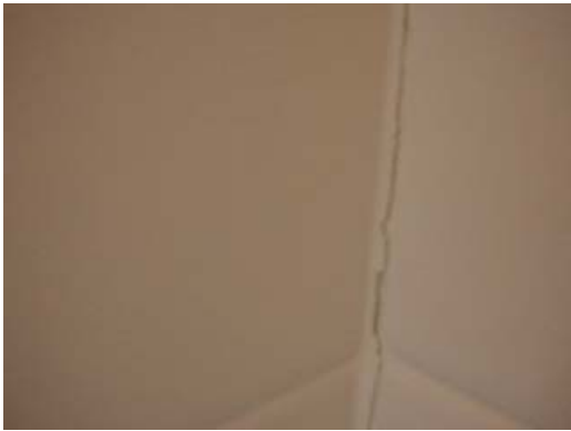
Cracking above the tile in bathtub enclosure.
