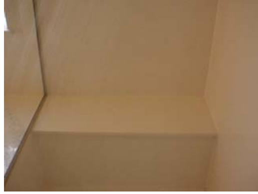
The sitting area located in the master bath shower stall should be monitored on a consistent basis for failure of sealant. At this time it appears to be in good shape but these areas are vulnerable to moisture intrusions.
