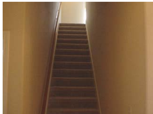
For Improved safety I recommend additional lighting for the stairway area.
