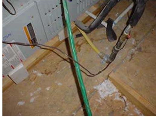
Data cable lines should be secured to allow better access to HVAC system.
