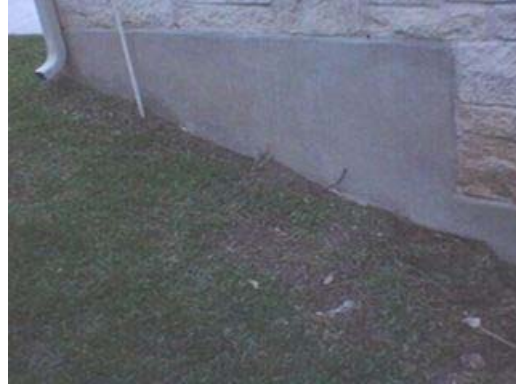
Evidence of erosion, recommend guttering be extended on both sides of the house.
