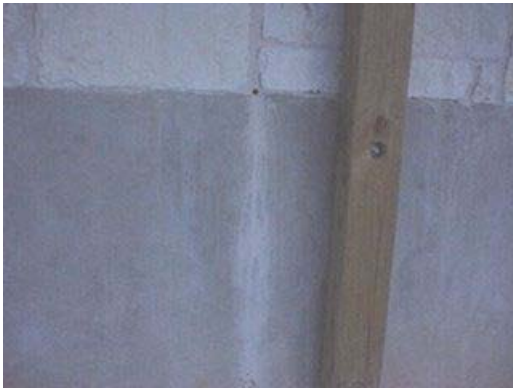
Evidence of excessive moisture flowing out of weep holes.
