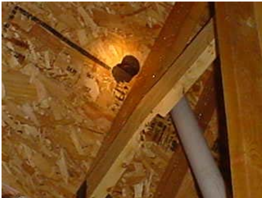
Note - Collar tie severely notched causing failure of the framing member, should be repaired. Also hole in roof decking should be repaired.
