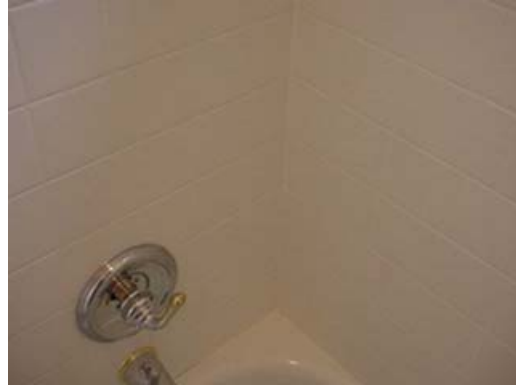
Re-caulk the bathtub tile enclosures.
