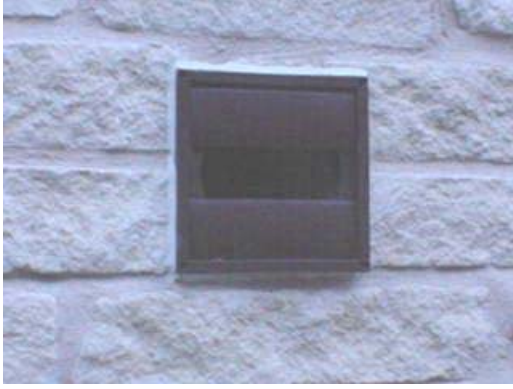
Vent cover missing back draft panel, should be repaired.
