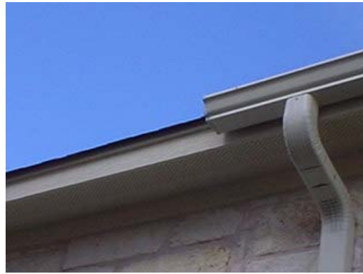
Recommend the extension of the gutters to include the entire side of the house or at least protecting the electrical service panel.
