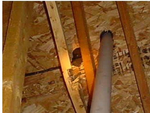
Hole in roof decking and collar tie severely notched causing damage, this should be repaired.
