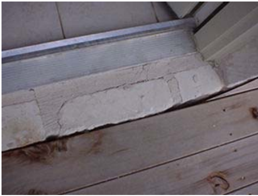
Cracking and loose mortar at the doorsill should be repaired.
