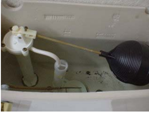
Minor adjustment needed to back bathroom toilets valve. Toilet runs on, this should be repaired.
