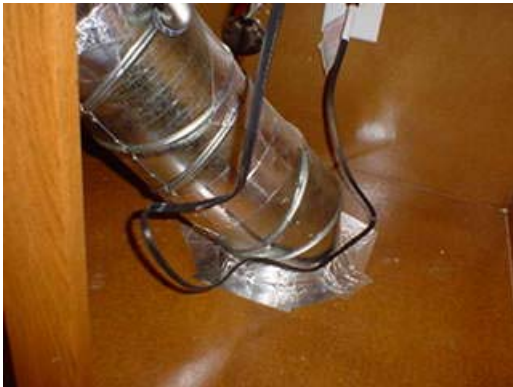
Electrical wiring in contact with flue vent, located under cabinet in kitchen.
