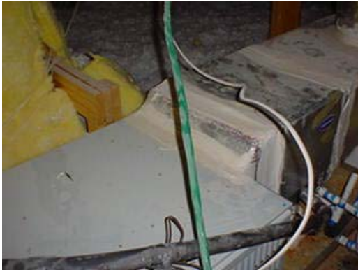
Loose wiring should be better secured and protected.
