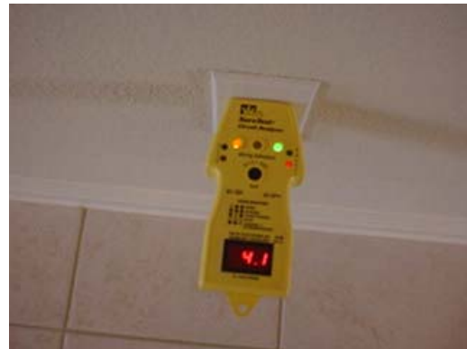
Reversed Polarity receptacle located in the front entrance hallway.
