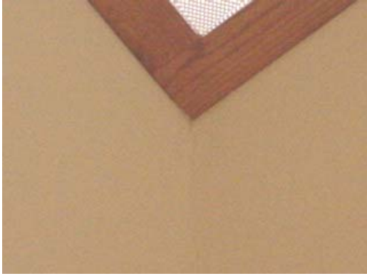
Sheetrock cracking in skylight area
