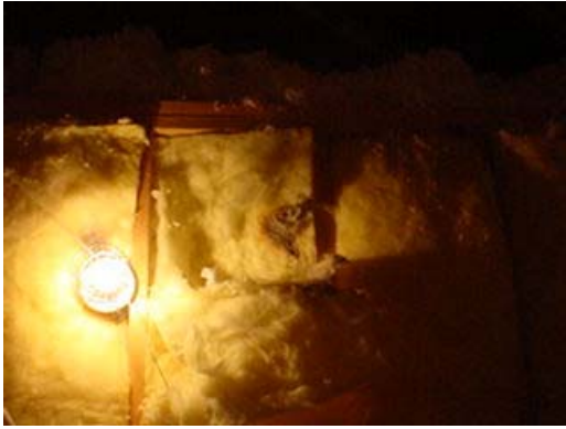
Incandescent light considered to be too close to combustible materials and should be repaired.
