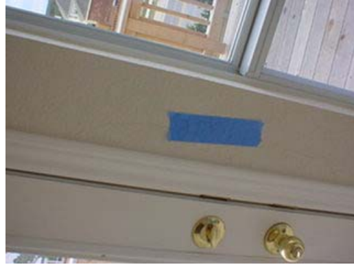
Moderate cracking of sheetrock due to expansion and contraction and /or settlement of framing members. This should be repaired.
