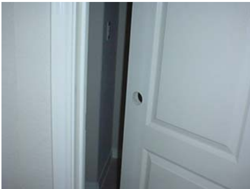
Missing Door Hardware for half bath.
