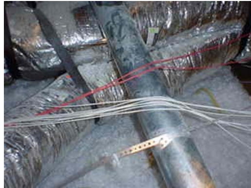
Communication wiring touching heater flue vent, wiring should be rerouted as to not being in contact with heater flue vent.
