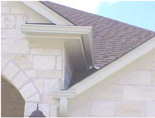
Down spout to shingles, This causes premature deterioration of the shingles.
