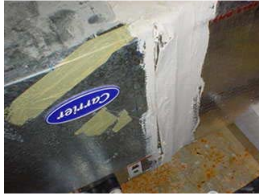
Seal has been cut on the HVAC unit - this should be repaired.
