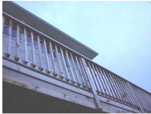
Railing considered loose, should be repaired for safety.
