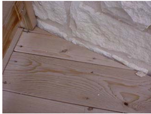
Back decking board is not secured properly this should be repaired.
