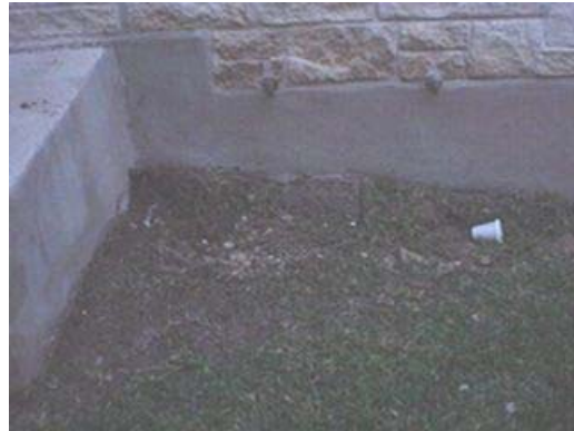
Erosion already taken place.
