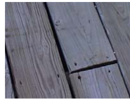
Loose decking- trip hazard. Repair needed.
