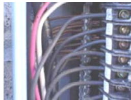
Wiring crowded on bus bar
