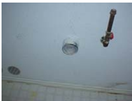
With two 90 degree turns dryer vent suspected to be too long.
