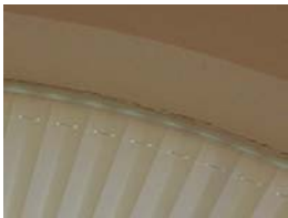
Window needs re- sealing
