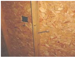
Hole in roof decking
