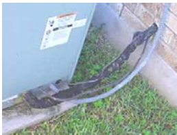
Insulation for refrigerant piping needs replacement
