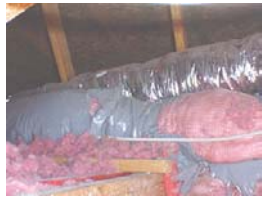
Old gray flex ducting shows evidence of attic overheating
