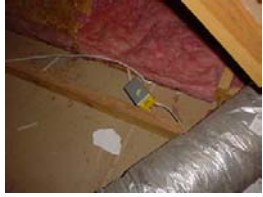
Junction box not secured
