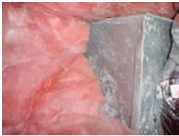
Air supply box needs insulation
