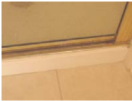
Shower door bottom seal needs repair
