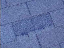
Missing shingles
