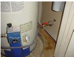
Gas piping for water heater should have sediment trap
