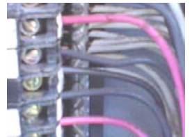
Wiring crowded on bus bar
