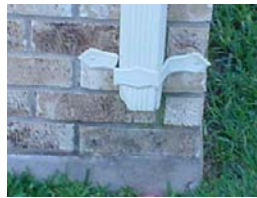
Downspout tail missing
