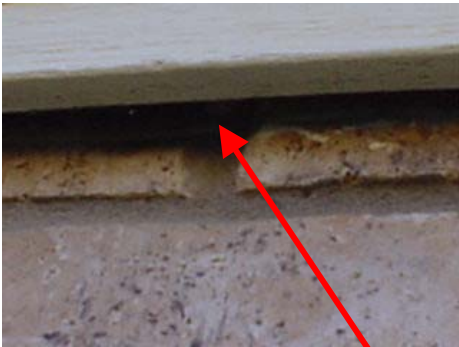
Openings where brick and siding meet should be sealed.
