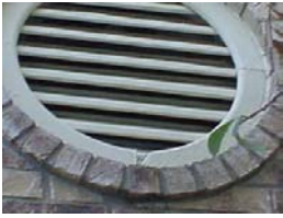
Water damage to vent cover
