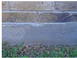
Slab re-faced- small crack
