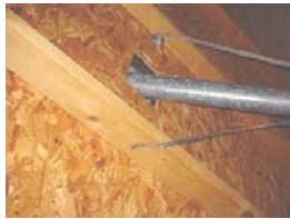
Water heater flue vent in contact with combustible
