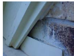
Water intrusion behind flashing
