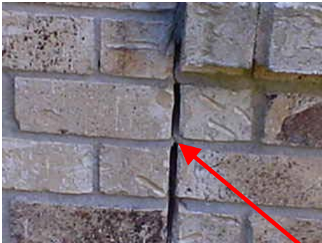
The expansion joint should be filled.
