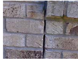
Expansion joint should be filled
